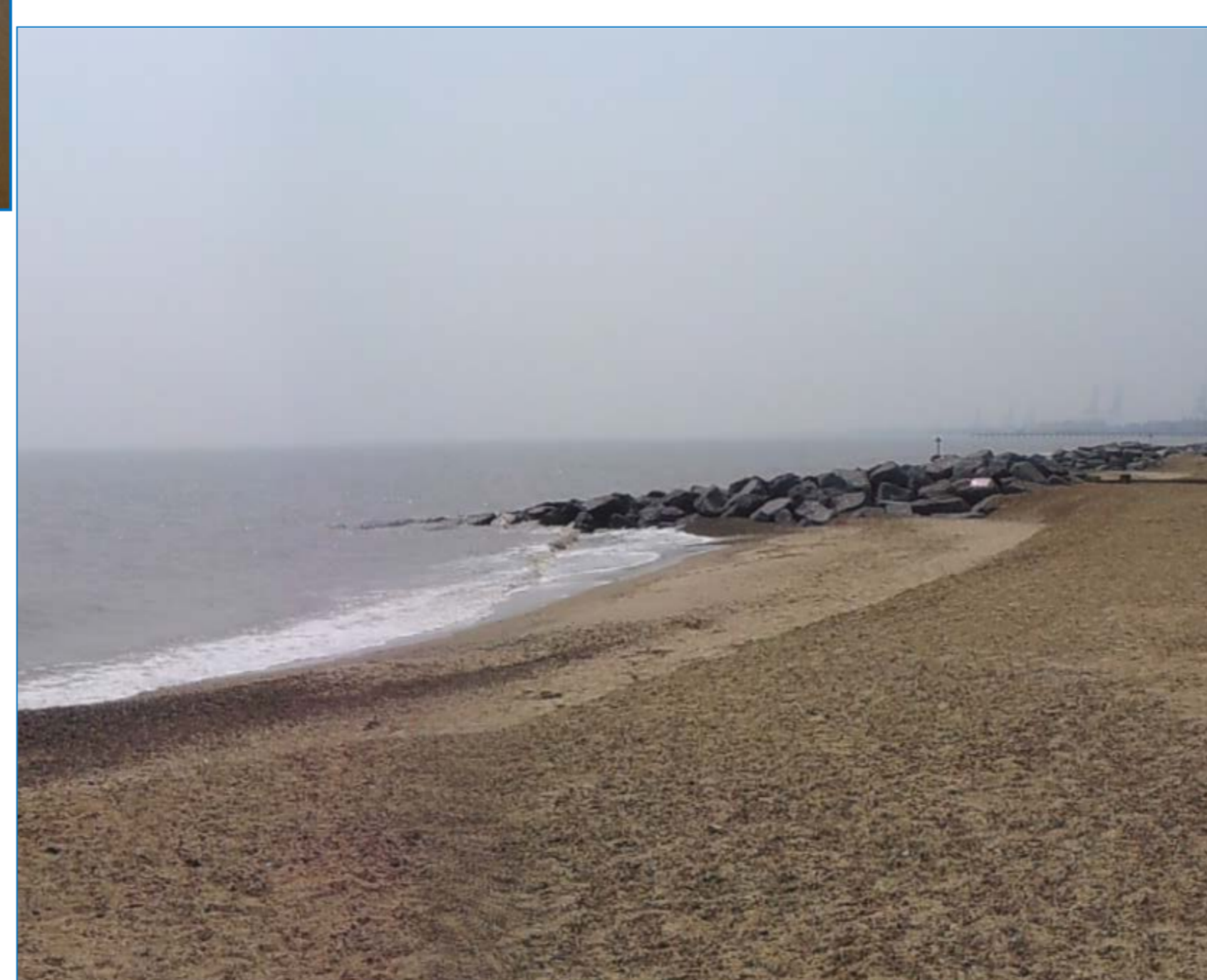
Recently Recharged Beach at Felixstowe – similar sourced material to the Clacton and Holland-on-Sea frontage
