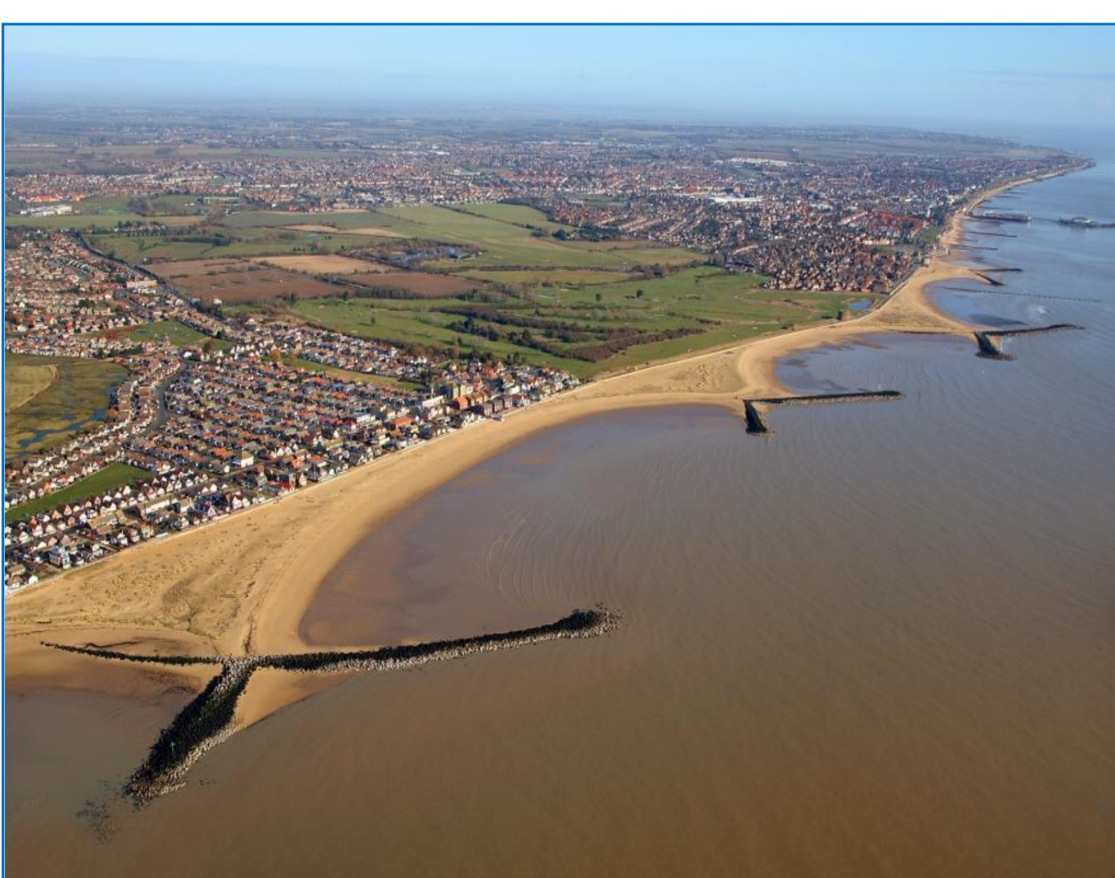
Fishtail rock groynes at Jaywick
