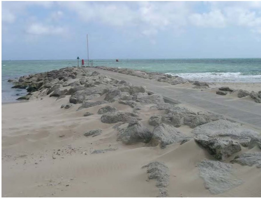
Figure 2-8 Flat concrete walkway on top of a rock groyne at Poole (18/05/2009)
