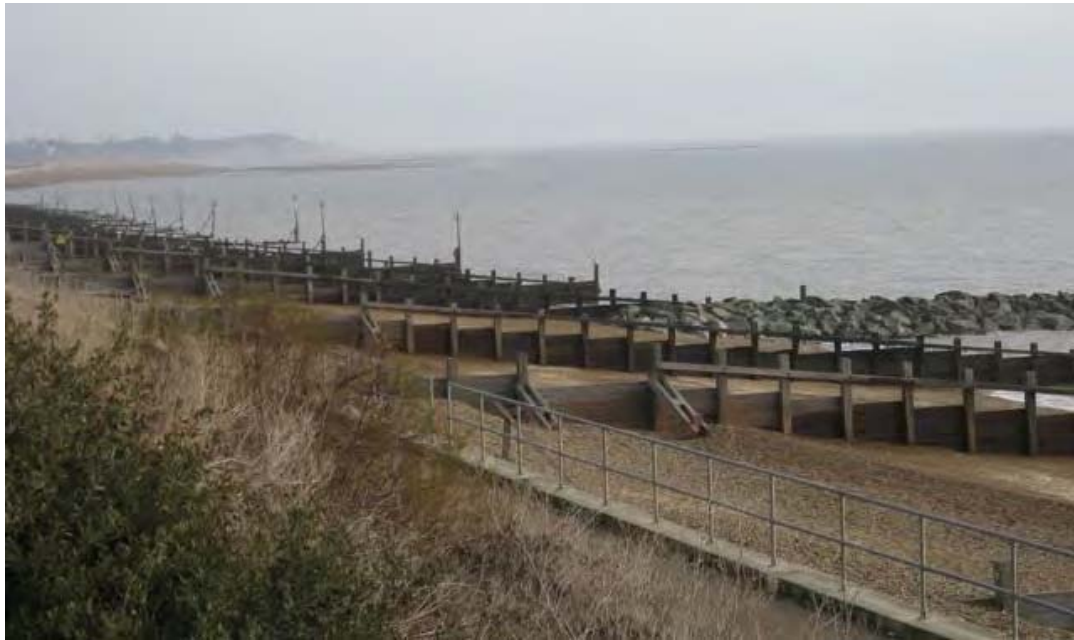
Figure 2-17 Timber groynes in the distance with Hybrid groynes in the foreground at Brackenbury (February 2009)
