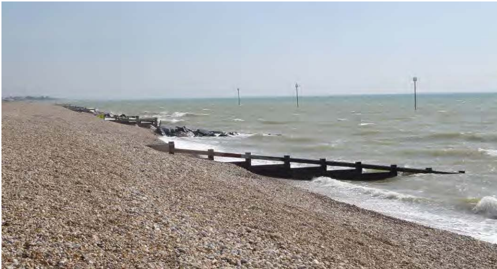
Figure 2-21 Hybrid groynes at Bognor Regis (May 2009)
