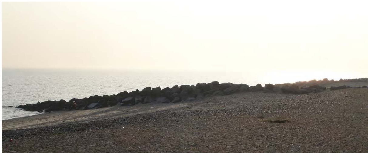
Figure 2-9 Rock groynes at Jaywick (May 2009)
