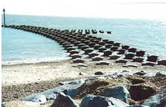
1 st October 2000 Following the completion of the scheme
