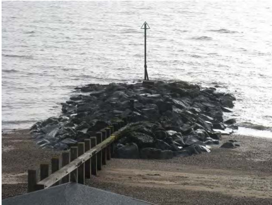
Figure 2-6 Hybrid groyne at Brackenbury, North Felixstowe (February 2009)
