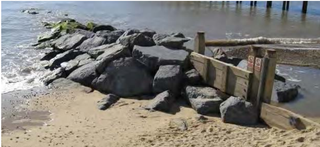
Figure 4-1 Closely spaced rocks preventing large voids in the rock groynes
