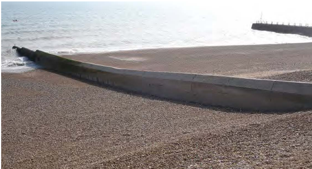
Figure 2-19 Concrete groyne at Brighton beach (May 2009)
