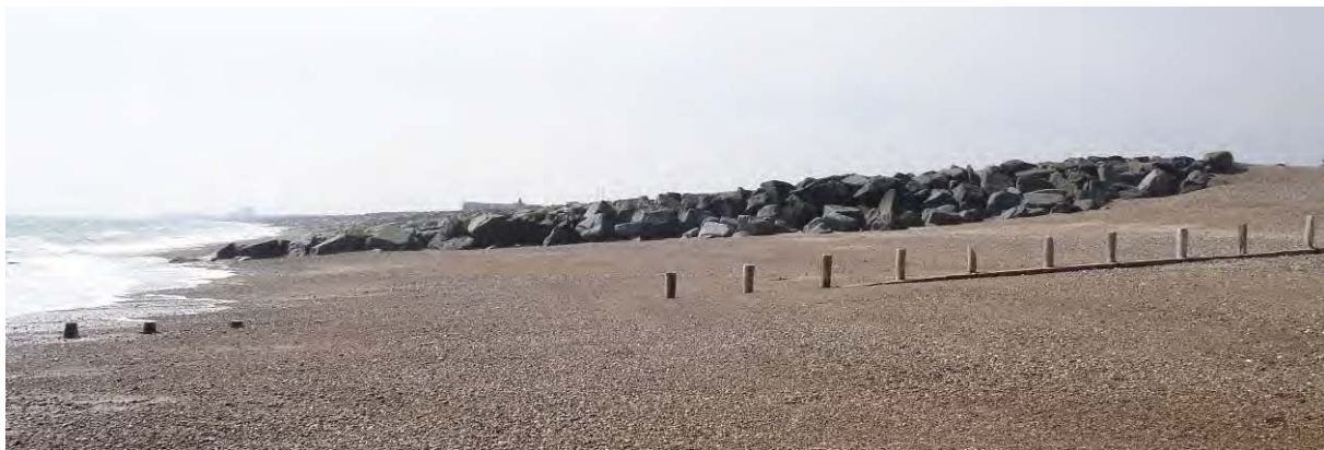
Figure 2-22 New rock groynes constructed alongside timber groynes at Shoreham-on-Sea (May 2009)
