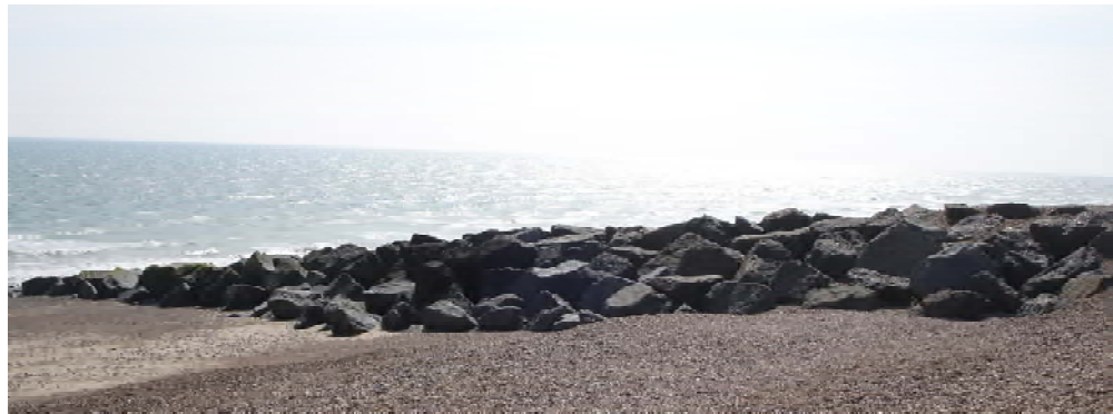
Figure 2-3 Rock groyne at Shoreham-on-Sea (May 2009)
