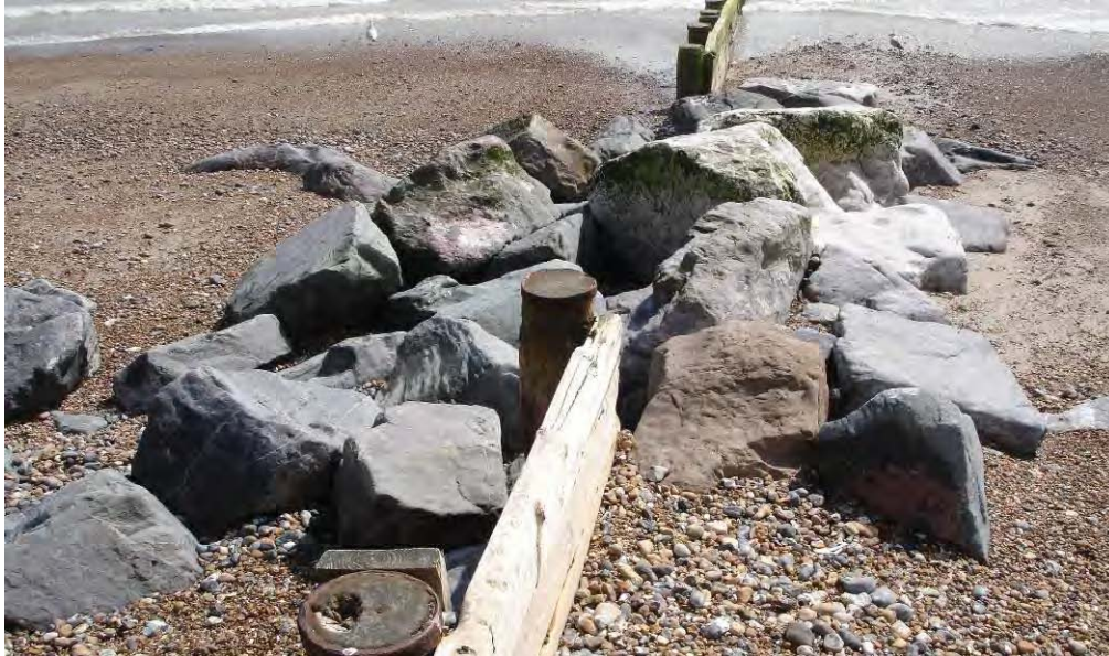
Figure 2-23 Repairs to a timber groyne at Worthing (May 2009)
