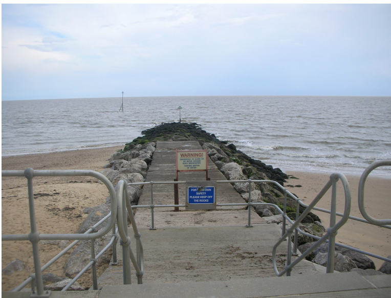
Figure 22: Higher Sand North Groyne 84
