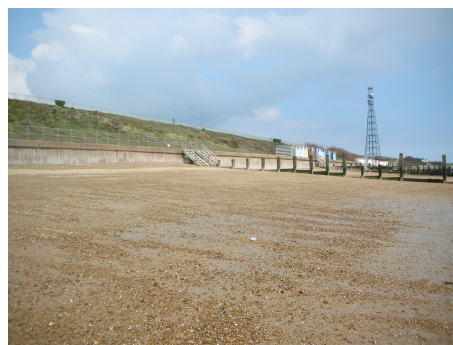
Figure 14: Holland Groynes Fill c
