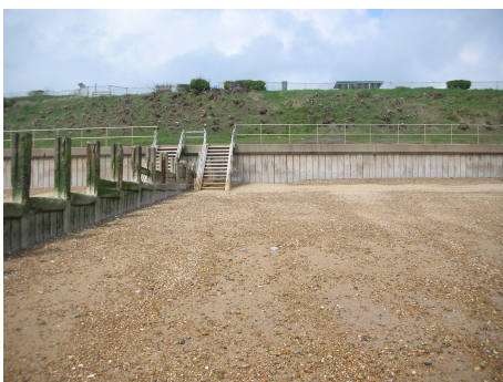
Figure 13: Holland Groynes Fill b
